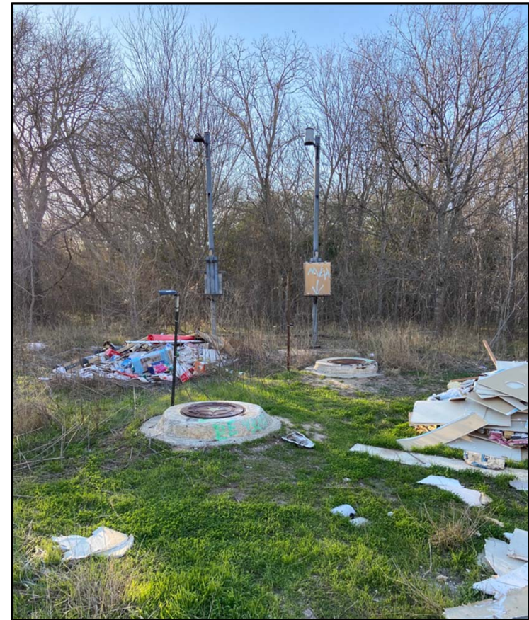
Downstream MH 1-1 Near Adjacent CIPP Project (Facing West)
